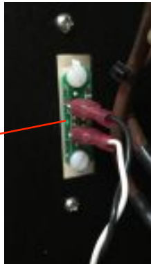
Flow transducer wiring
